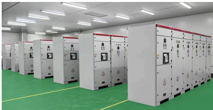
MNS低压智能配电柜 MNS low-voltage intelligent distribution cabinet
