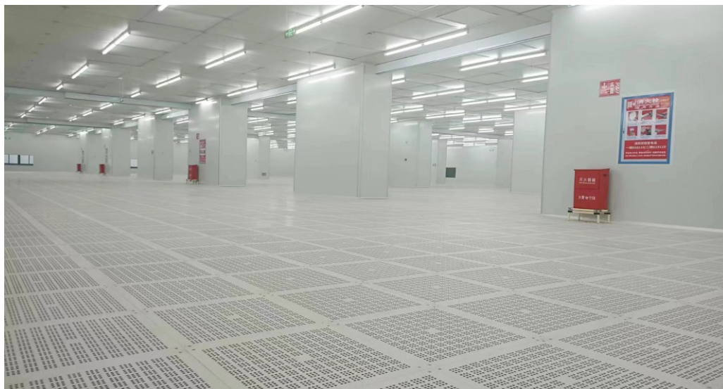
洁净室, 铝合金架空地板 Cleanroom, ISO class 6, Aluminum alloy raised floor
